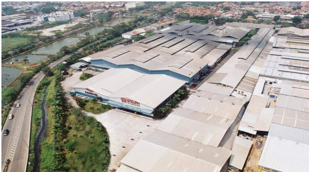
Kapuk Plant (Radiator Facilities)
